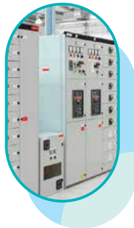
MCC Panels (Motor Control Centre)
